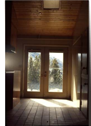
Thermal mass flooring
