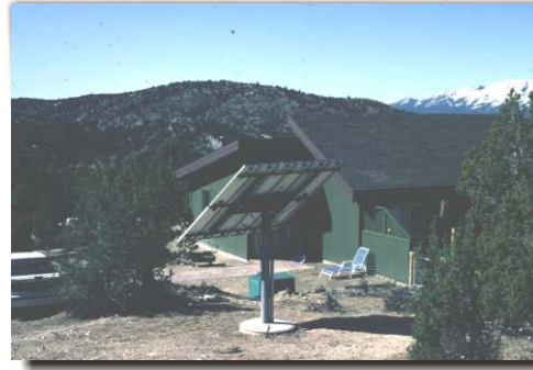
PV panels provide clean power
