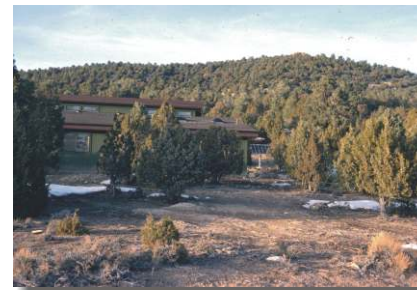
View from the South side
