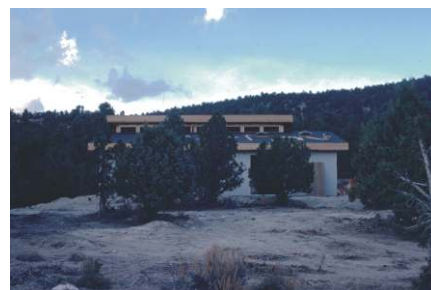
Building wrap & fascia
