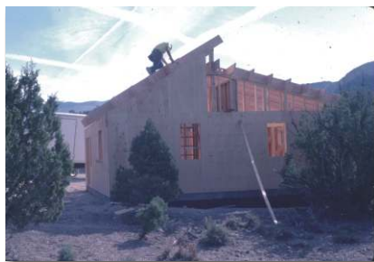
2 X 12 Roof rafters.
