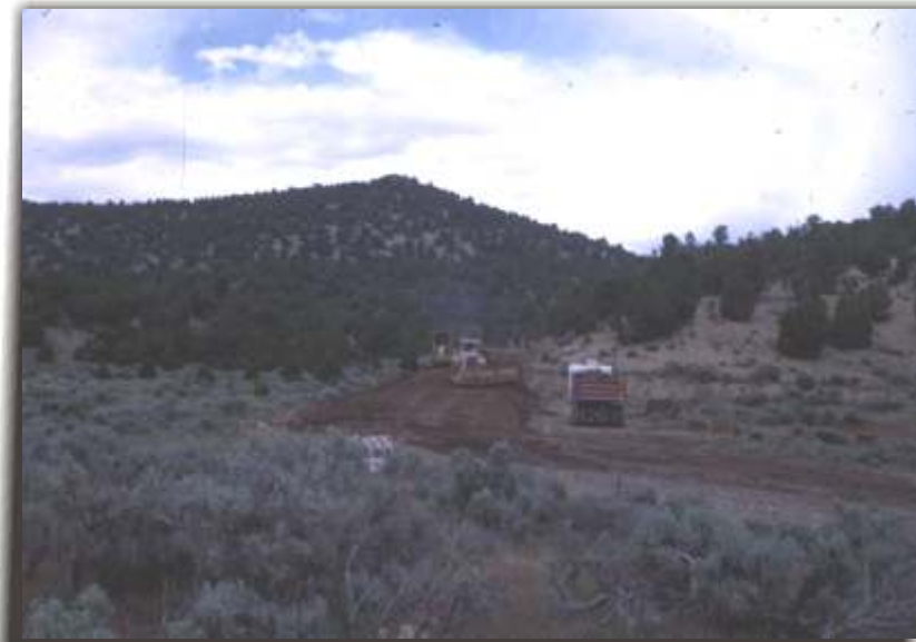
Access road clearing and grading.
