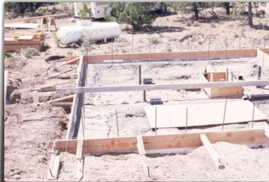
Comfort station perimeter forms layout.
