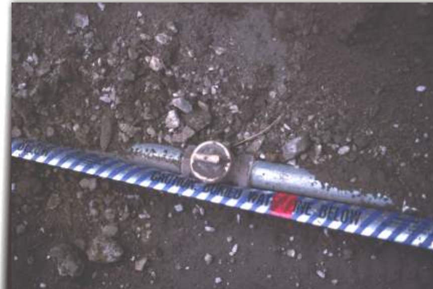
Waterline , valve, and locator tape installation.
