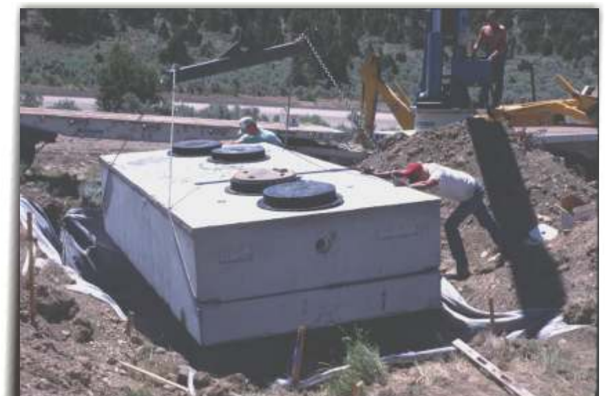
2500 gallon septic tank being set in place.
