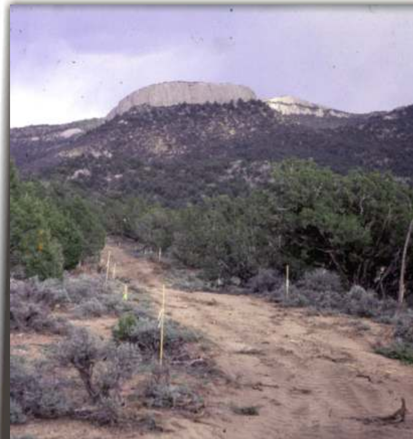
Road alignment along natural contour.
