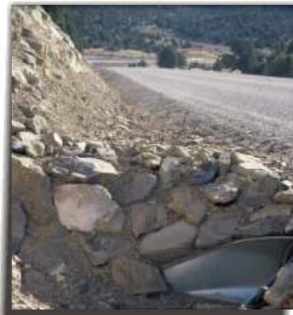
Hand-fitted stonework at culvert
