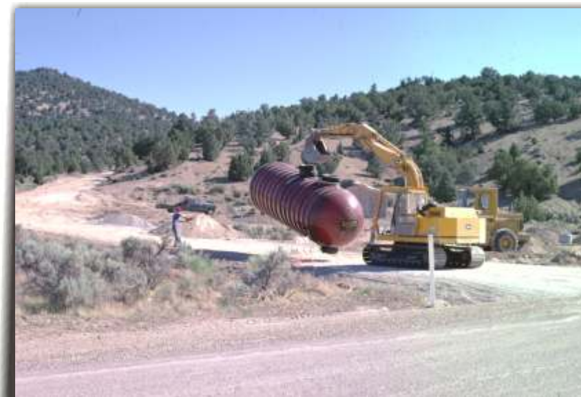
Potable water storage tank traveling to installation site.
