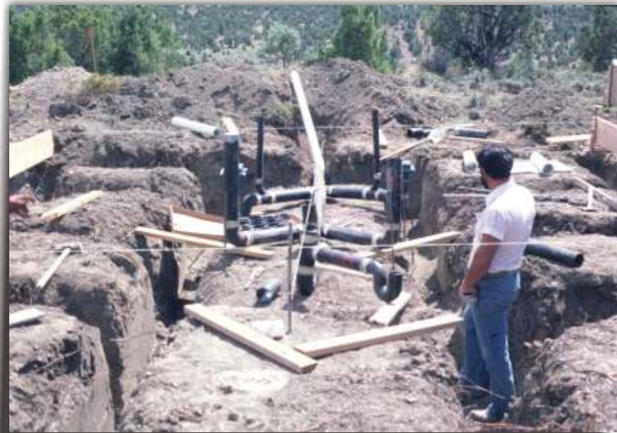
Comfort station excavation & plumbing installation.
