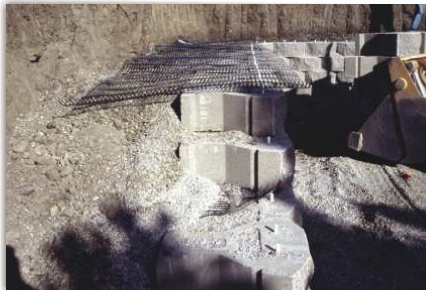
Geogrid placement in Ret. Wall
