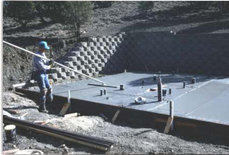
Finishing Slab on grade
