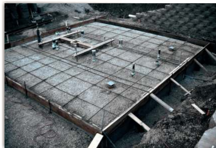
Slab block-outs and reinforcements
