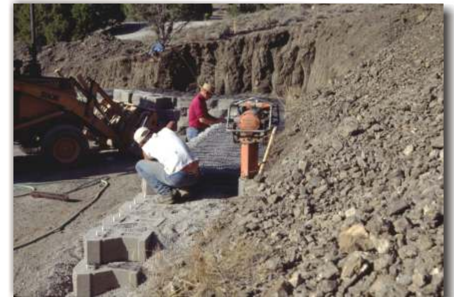
Modular Block retaining wall construction
