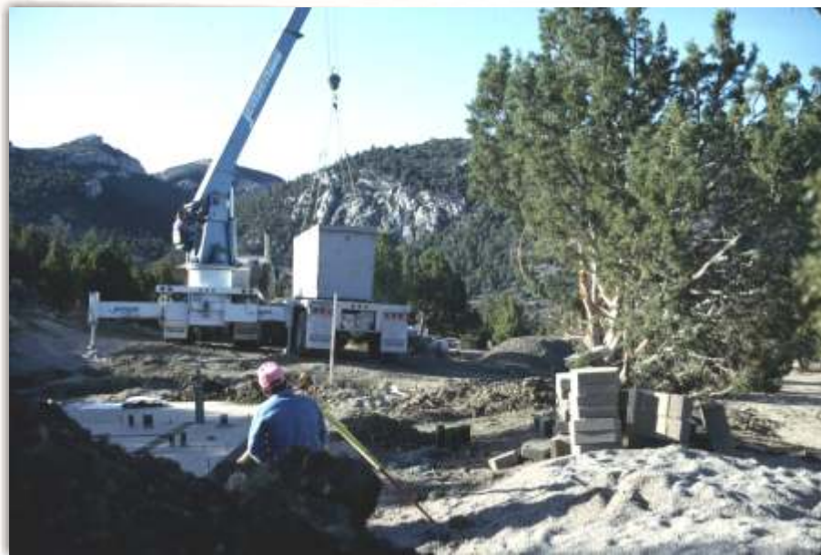
Septic Tank installation
