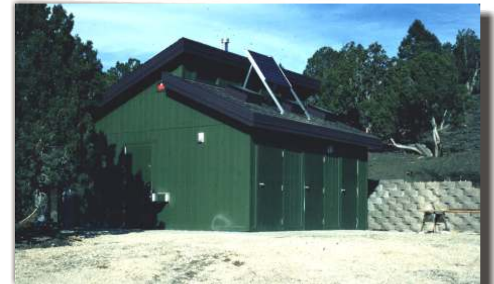
Solar PV Panels on completed Comfort Station
