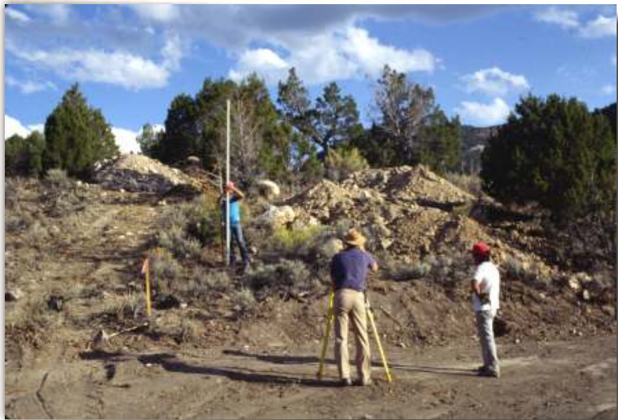
Setting grade for drain field trenches & pipe
