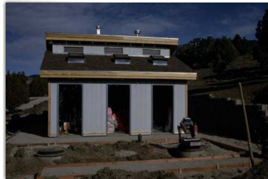
Interlocking Paver base preparation
