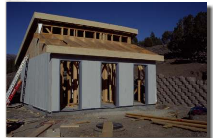
Roof Framing & Siding
