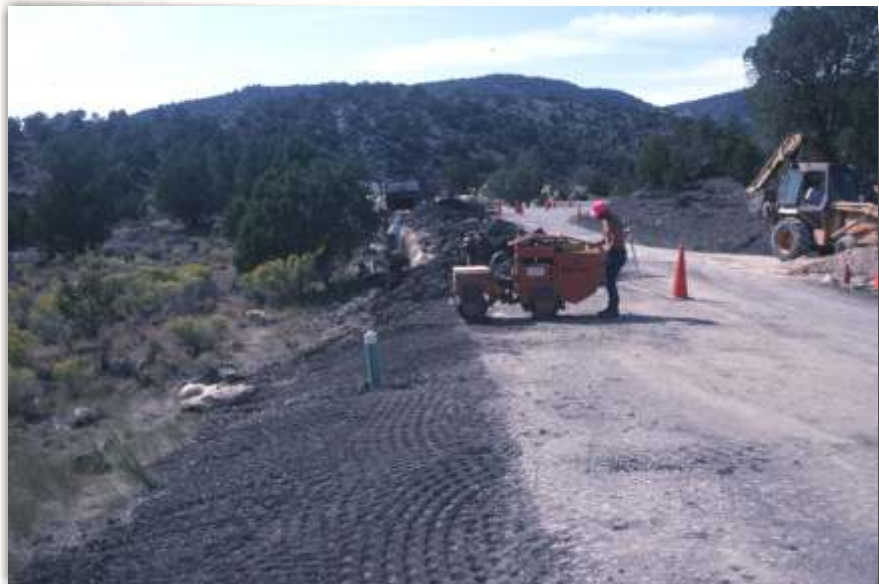
Sewer line finish grade/compaction
