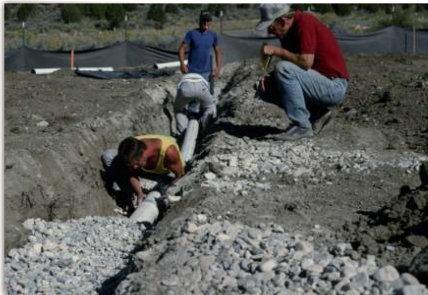
Pipe & cover rock installation
