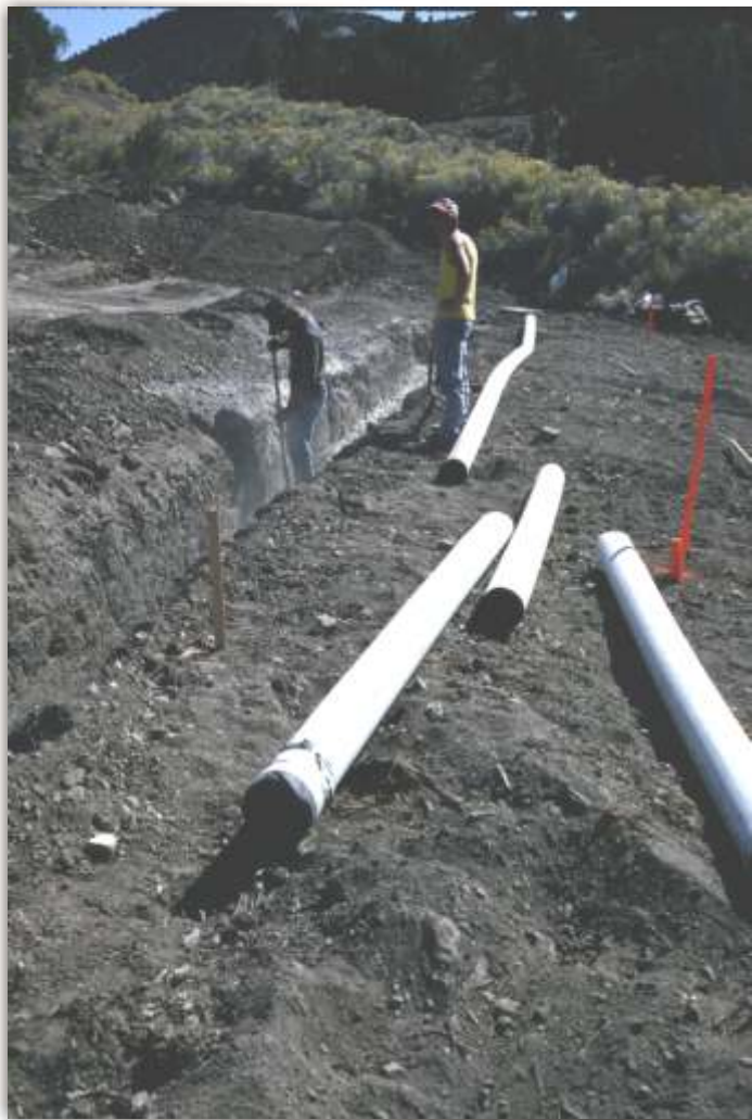
Drain Field rock & trench installation
