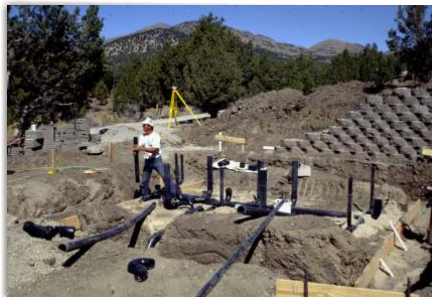
Rough plumbing installation
